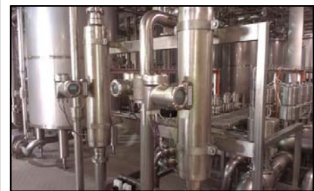
OPTIMASS includes entrained gas management feature and provides full transfer with accuracy of 0.4% or better
